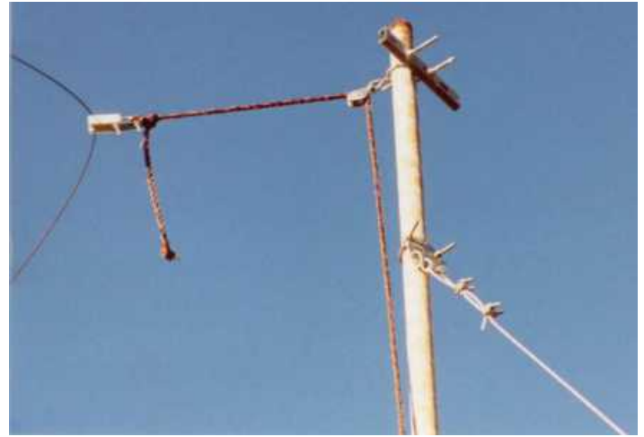
Figure A: Detail of a Mast Support
